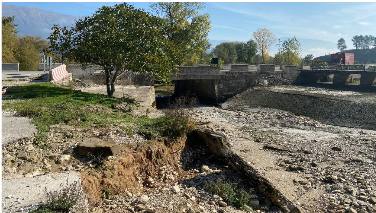
Figure 11: Images of Viroi Bridge
